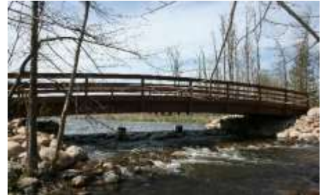
Bridge over the Turtle River
