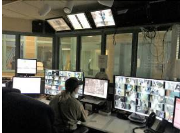
One of two Control Rooms
